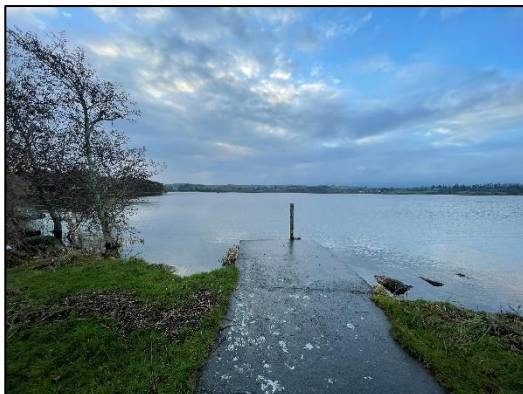
Plate 3-7 Existing slip into Lough Rea which will be upgraded.
