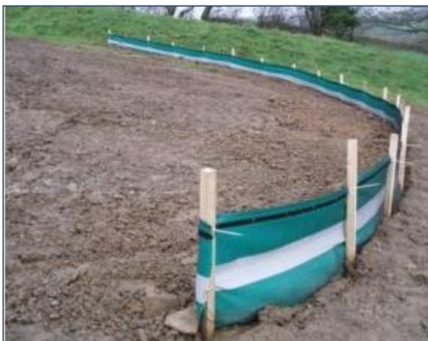
Plate 3-4 Embedded Silt Fence
