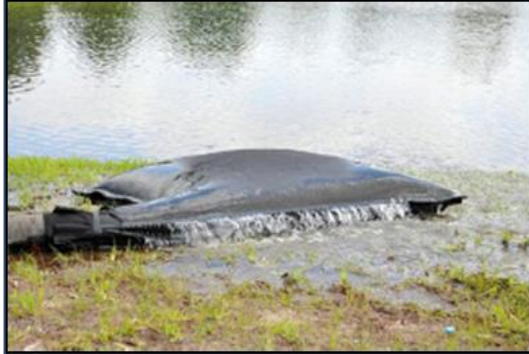
Plate 3-1 Silt Bag with water being pumped through.
