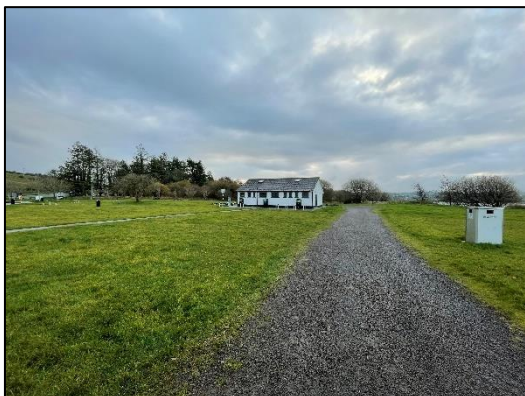
Plate 3-5 Existing toilet block to be demolished within the Proposed Development site
