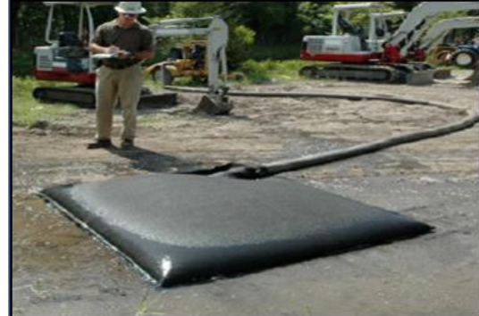
Plate 3-2 Silt Bag under inspection
