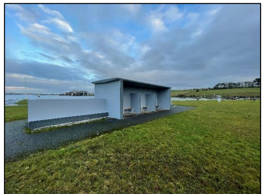
Plate 3-6 Existing changing shelter to be demolished within the Proposed Development site
